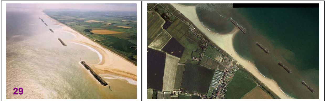
Tombolos forming behind offshore breakwaters at Sea Palling, Norfolk.
